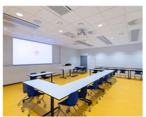
speeches. Stouenborg flush mounted Meyer Sound UP-4Slim loudspeakers in the ceiling. A Panasonic projector is also installed in the ceiling and fires onto a tensioned roll-down screen. A touchscreen was installed as well as Wolfvision Cynap.
