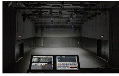
Above top: MOVEKET hoists and Elion load cell system provide the structural flexibility required for Dansehallerne's main performance space.
