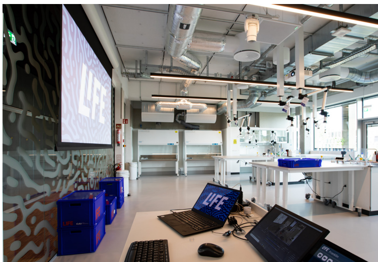
One of the teaching laboratories [left] and the main rack room
